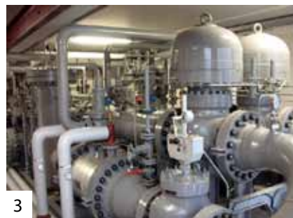
3 Detail engineering of CO 2 measuring and regulation stations which led to standard sales contracts for a major CO 2 distribution network in the Netherlands.
