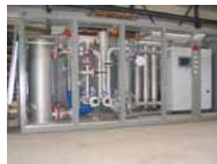
TCR under construction
